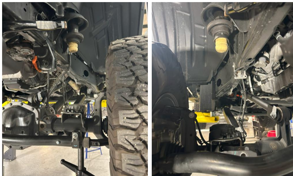
Figure 1: Axle supported, and spring removed (track bar removed)
